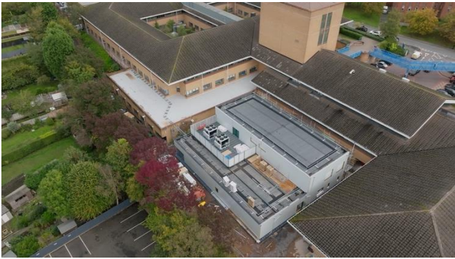
Cannock Chase Hospital Community Diagnostic Centre
